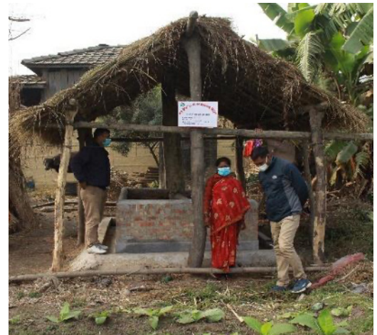
Vermicompost Pit Constructed
